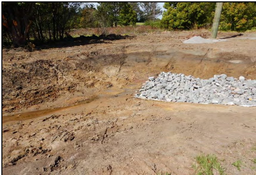
Photo 14: Cutting of about 1.5 m depth with orange brown silty clay exposed
