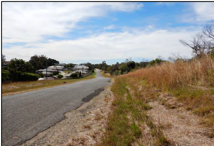
Photo 16: Possible cut on eastern side of road with embankment fill on left
